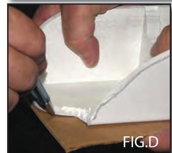
STEP3- After making the necessary modifications, place the threshold back into the shower to ensure all modifications are correct and dry fitting the threshold is accurate.
